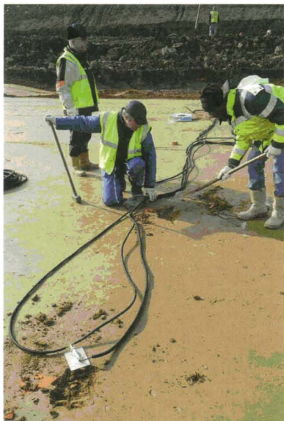
Instrumentation of the reference embankment built with treated soil as part of the TerDOUEST project.
