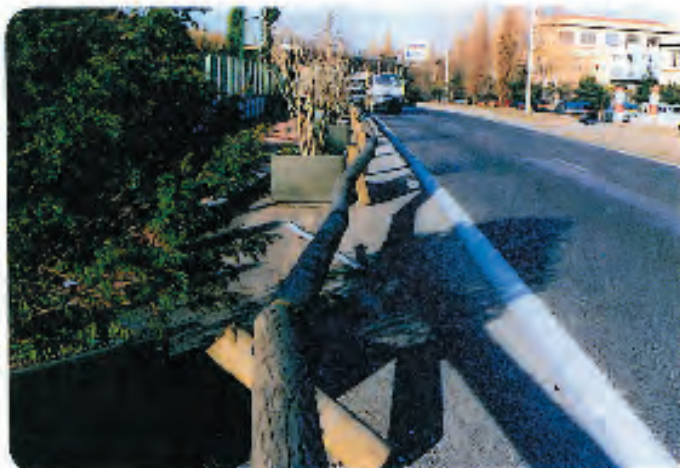
This wooden barrier prevented the planter from obstructing a vehicle
