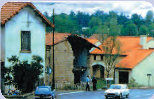
> House damaged by a heavy goods vehicle.
