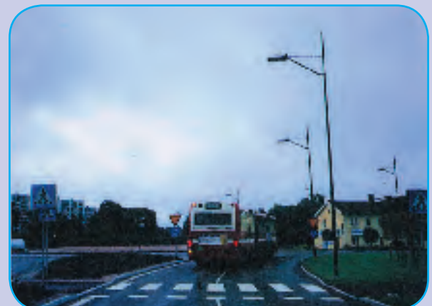
> Energy-absorbing deformable lamp-post. (Sweden)
