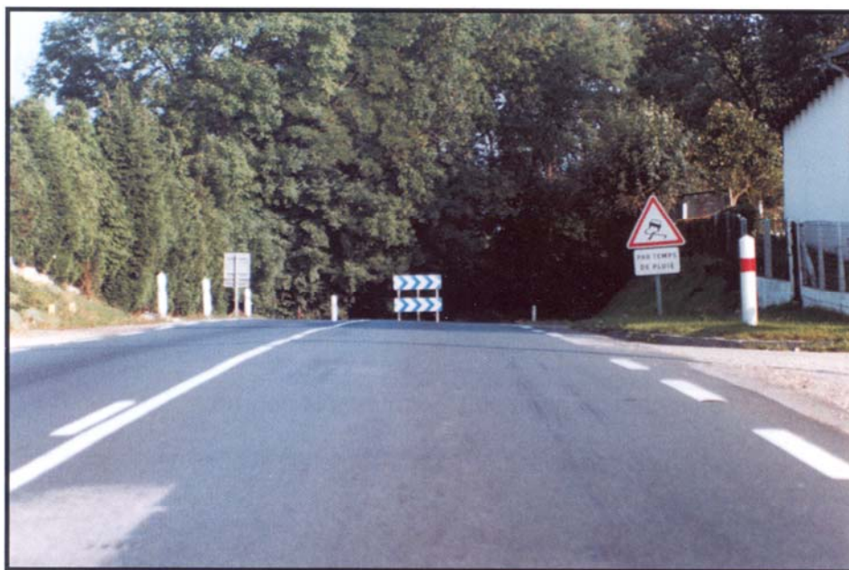
Late appearance of a bend immediately after a crest in the road
