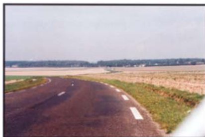
Danger at night!
