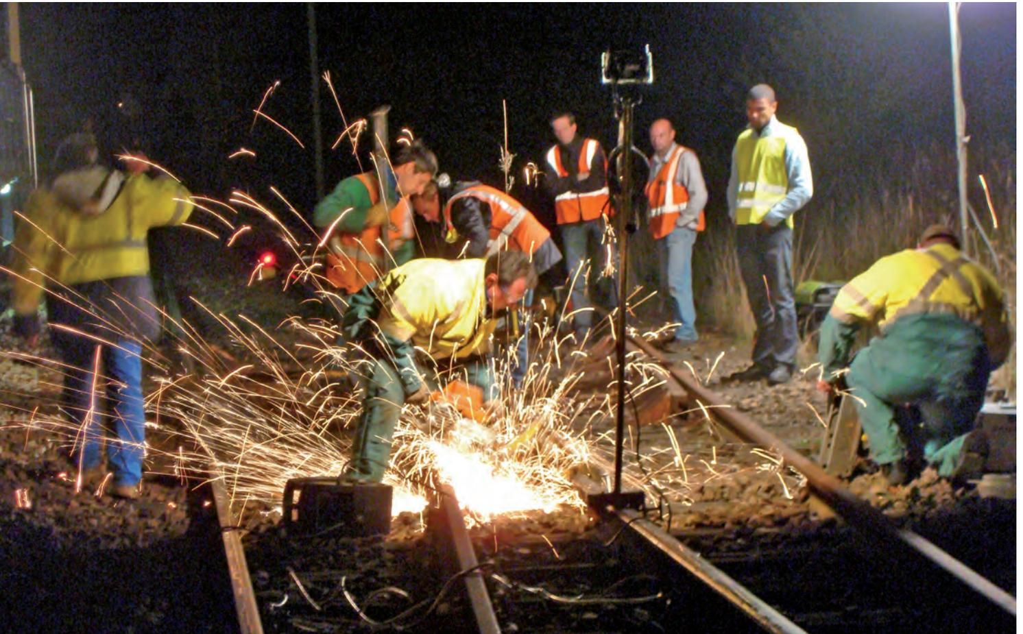
Rail-grinding during rail-switch replacement operations at night
